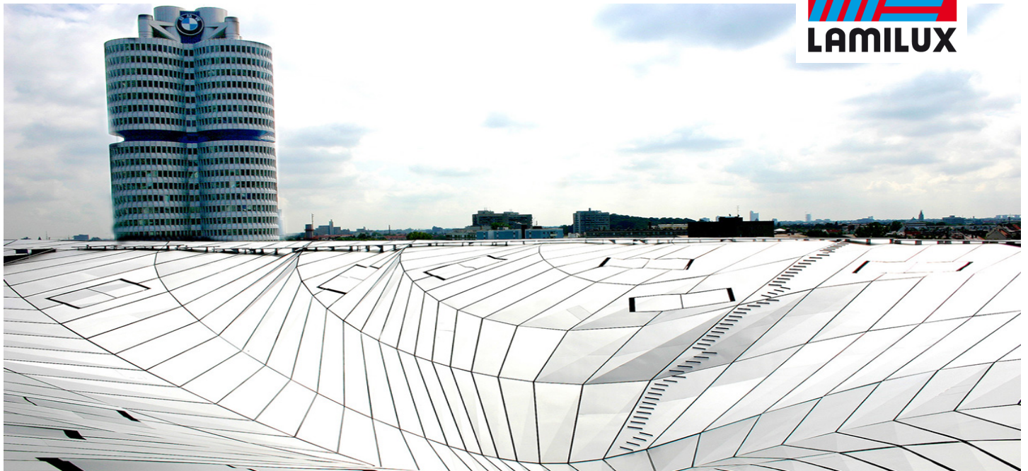
BMW Four Cylinder Building, Munich
